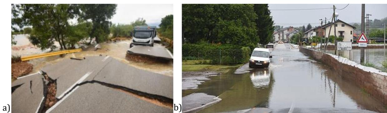
Figure 2-6 Examples of damages to transport infrastructure, a) Road damaged in flood in Zadar (Croatian Waters, 2018); b) flooded road in Karlovac (2019, <https://kaportal.net.hr/>)
