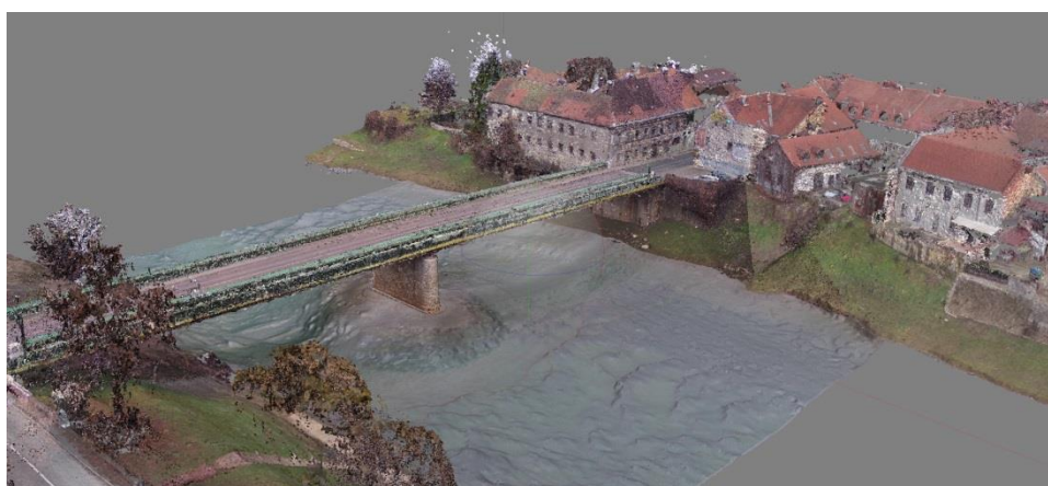
Figure 2. Point cloud of the Banija bridge with the riverbed (obtained from bathymetric inspection)
