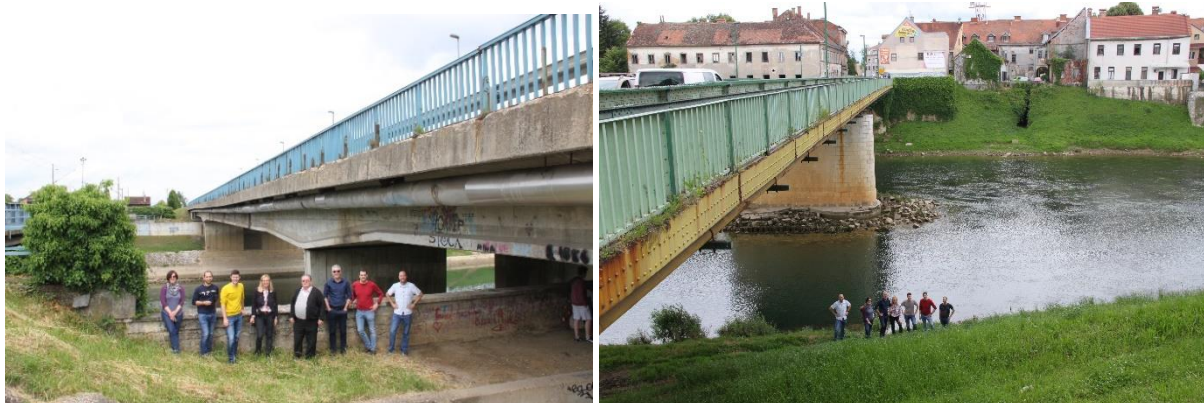
Figure 5: Consortium members next to the road bridge on state road DC 1 (left), and next to the Banijski road bridge (right)
